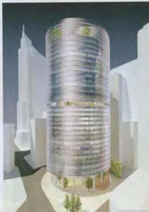
The double skin ventilated facade at 1 Bligh Street, a 31 storey building by Grocon and design by Architectus in association with Ingenhoven architects Germany.
