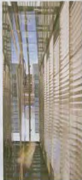
The double skin ventilated facade at 1 Bligh Street, a 31 storey building by Grocon and design by Architectus in association with Ingenhoven architects Germany.
